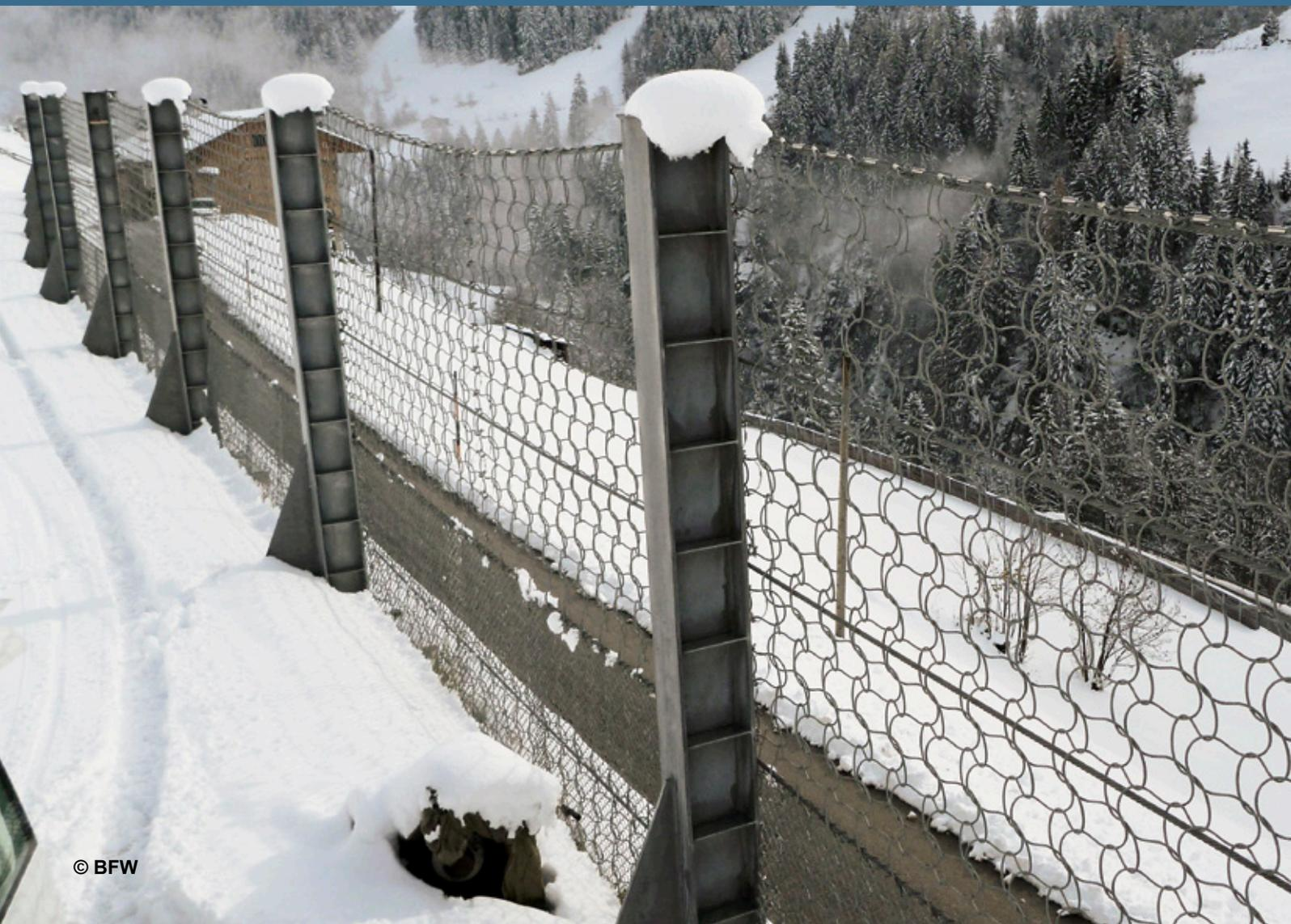
Snow catchment fences such as the SNOW-CATCHER do not prevent the initiation of avalanches but instead interact with an avalanche in the run-out or deposition zones in order to slow the avalanche and bring it to a standstill. This shortens the destructive reach of avalanches.
