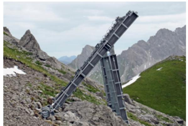
Compared to avalanche dams, catchment fences require less construction space. Thus, a larger area is available for the controlled interception and deposition of the avalanche.
