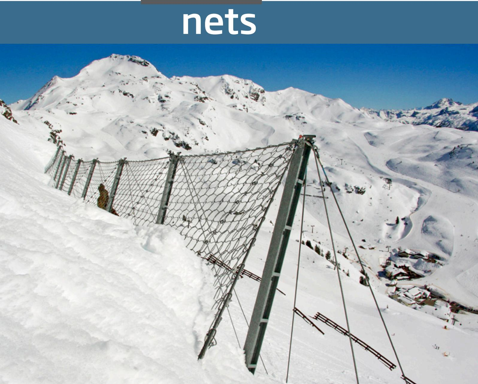
Snow nets prevent the development of avalanches by giving structural support to the snow mass in initiation zones having medium to large snow depths. This is in contrast to other approaches such as artificial release methods - e.g. by means of explosives – that initiate smaller avalanches before the hazard grows to an unmanageable size.
