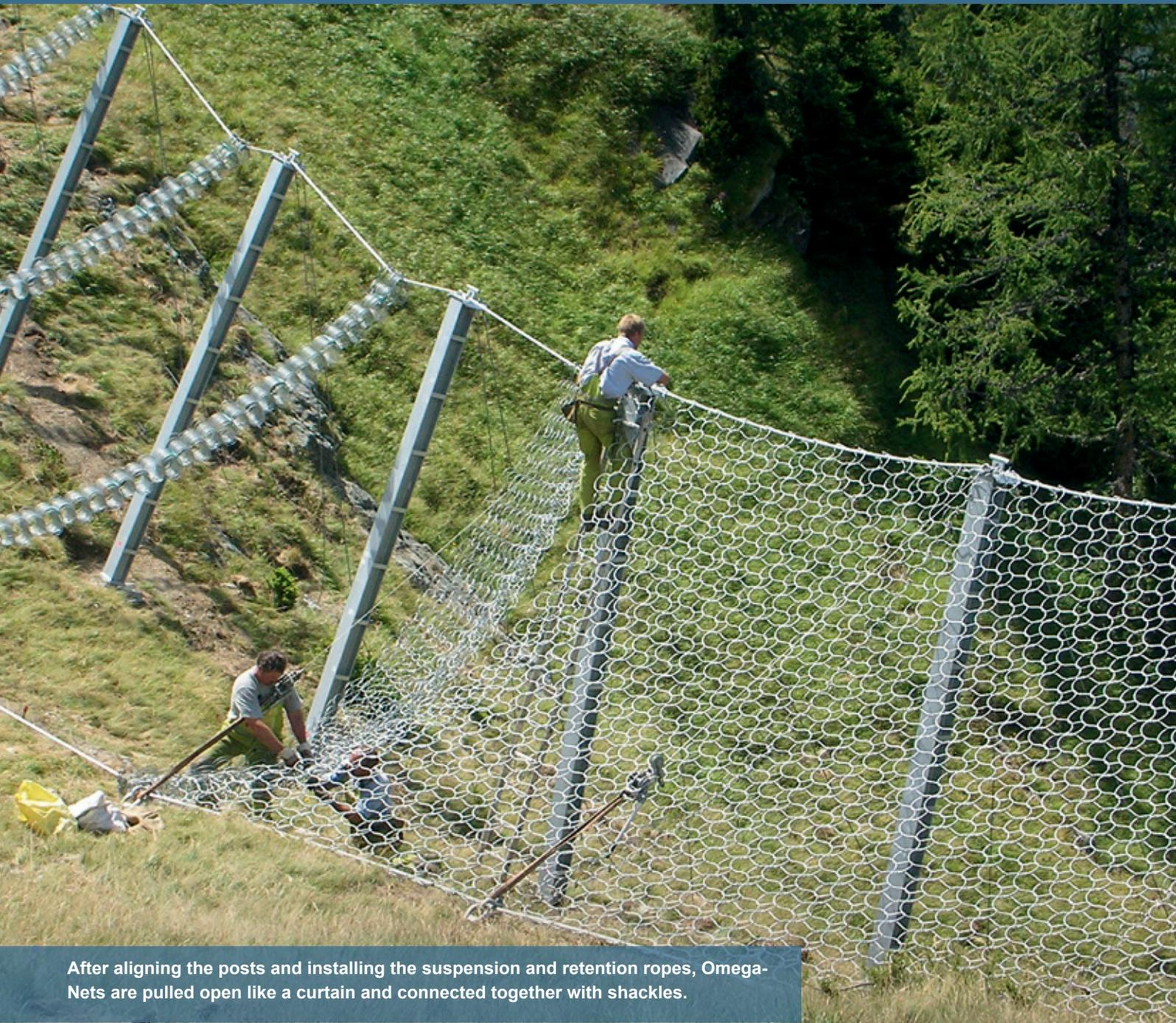
After aligning the posts and installing the suspension and retention ropes, Omega-Nets are pulled open like a curtain and connected together with shackles.
